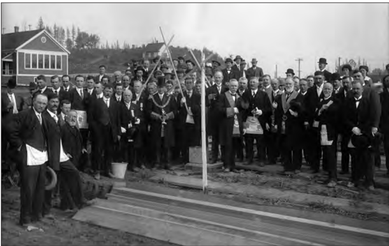
Laying the cornerstone of Abbotsford Lodge No. 70 Masonic Temple on May 18, 1912, MW Francis J. Burd, GM, officiating. —W. T. Cooksley, New Westminster
